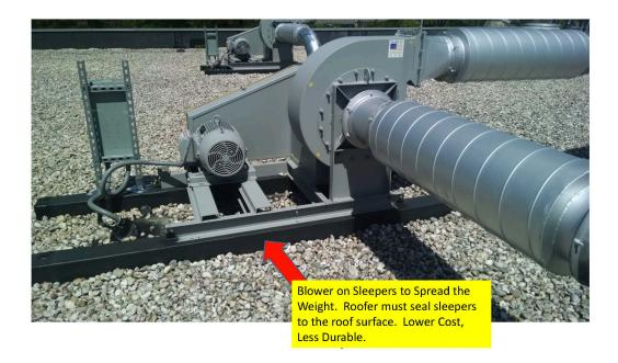
No matter what type of roof you have or how much weight the blower and support structure may add, Puhl always recommends consulting with your roof contractor and engineering company before any changes are made. These professionals will be familiar with the existing loads on the roof and can calculate what additional reinforcement if any will be required when adding weight to the roof system.
